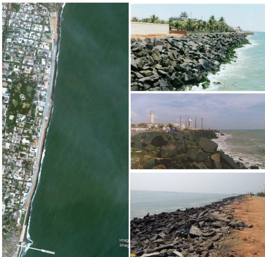
Figure 5. Constructed seawall along the Pondicherry coast
